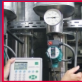
Testing a heating plant
